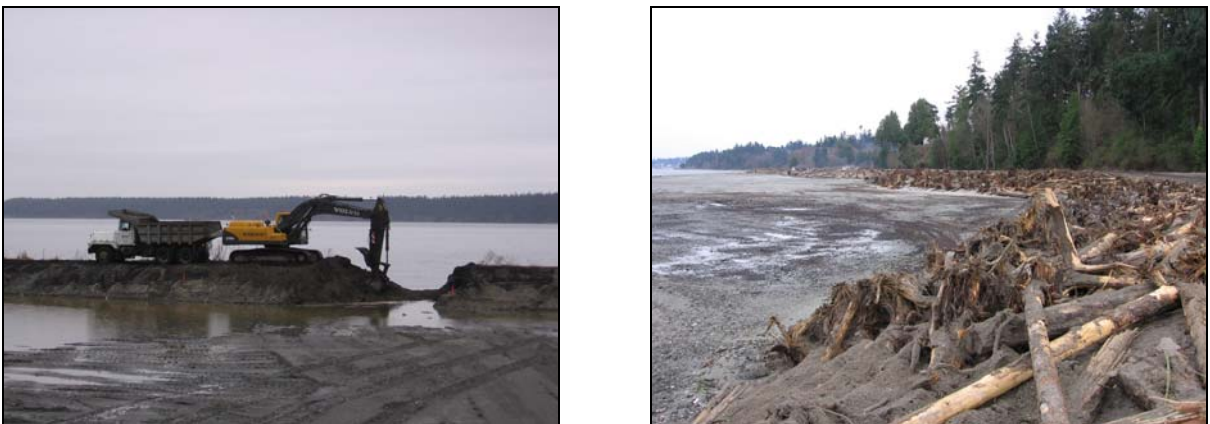
Figure 3. Photographs during and after work at the Chimacum/Irondale beach restoration site.
