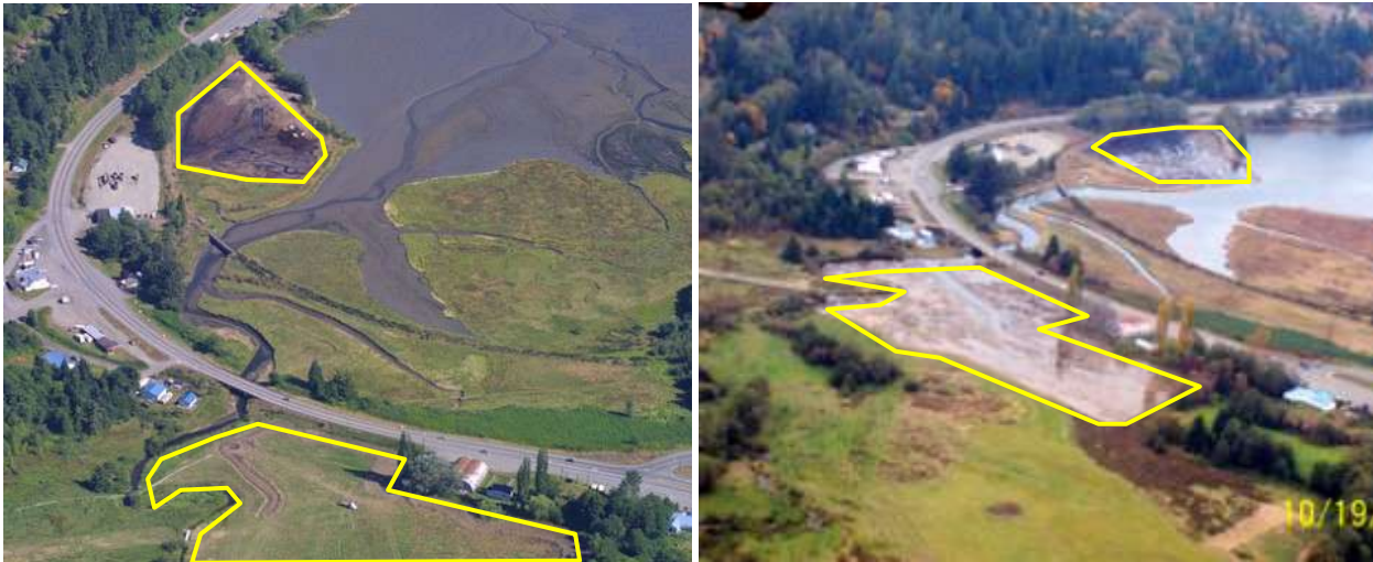
Figure 2.2: Salmon Creek estuary project aerial view during restoration (left) and after restoration (right).
