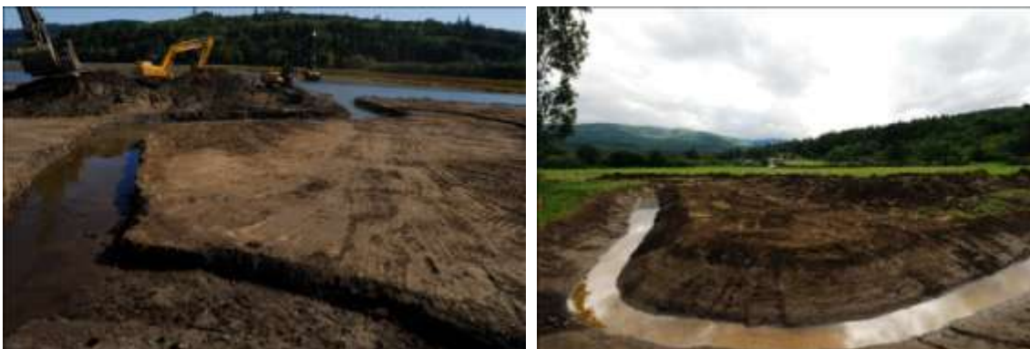
Figure 9.1: Tidal channel construction at Salmon Creek Estuary.
