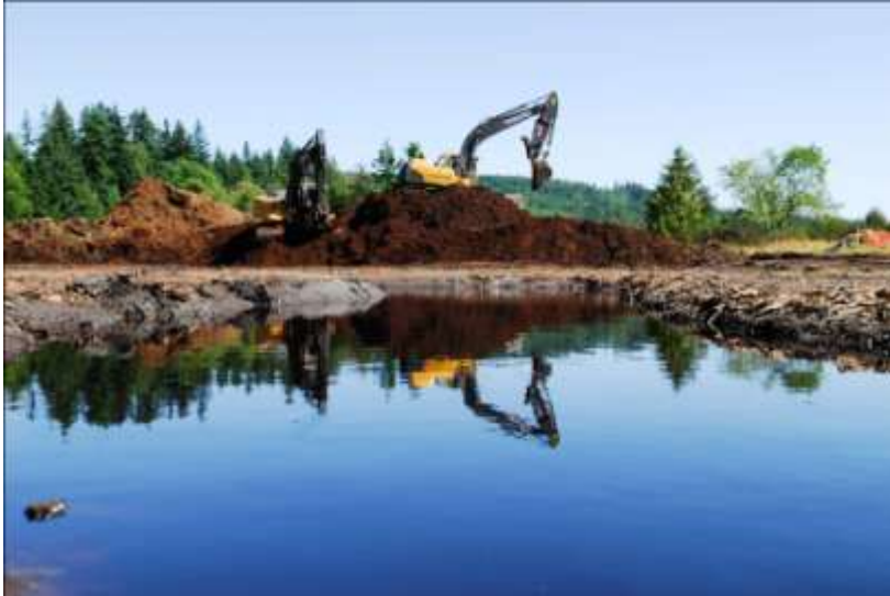
Figure 2.3: Excavation of the North Site Estuary, 2008 (Photo courtesy of NOAA)
