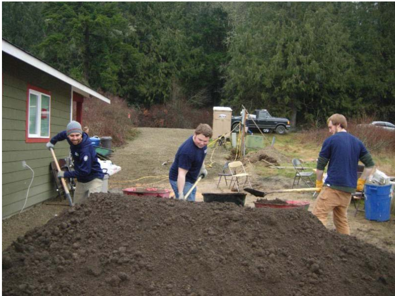
Working on a Habitat-for-Humanity home in Chimacum
