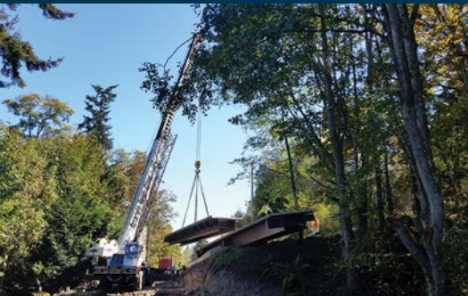
Crane positions bridge spans.
