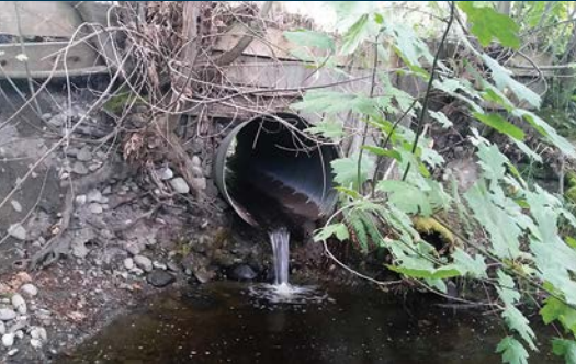
Perched culvert, a barrier to fish migration, on Matriotti creek.
