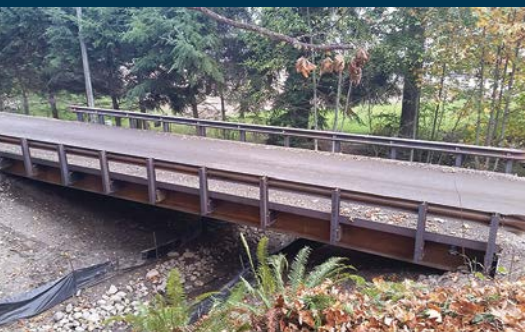
Steel bridge spans in place, ground re-contoured, and fish passage channel restored.
