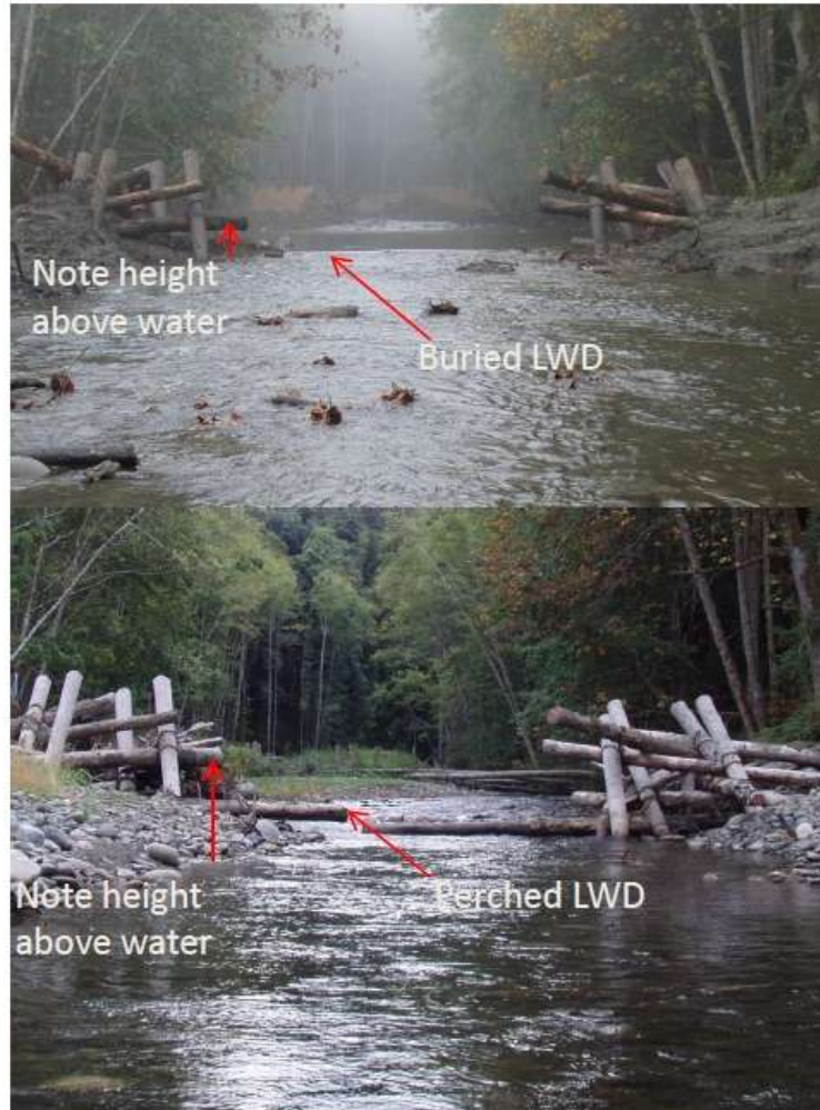
Figure 5.2. Photo depicting channel incision in the lower 50 meters of the new channel reach; top (2010) and bottom (2011).
